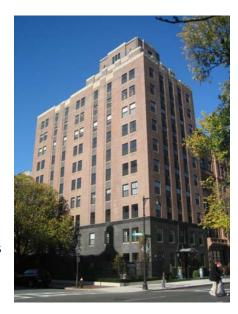
Toward that end, Abbot power washed the front and sides of the building, and selectively repointed the brick masonry surfaces.
